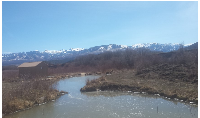
View of DCWC's infiltration gallery and pump station off Dallas Creek.
